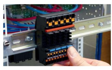
Push in jumpers for group supply (here: series connection of auxiliary contacts)
